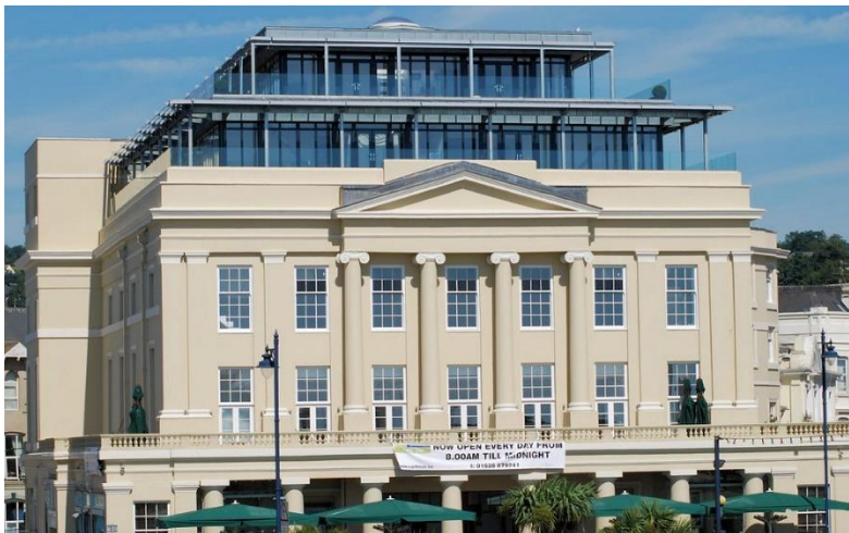
By August 2007 the new luxury flats had been built on top.
