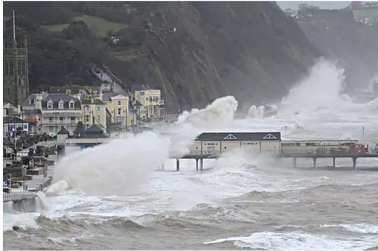
Pier and seafront being battered by storm waves.
