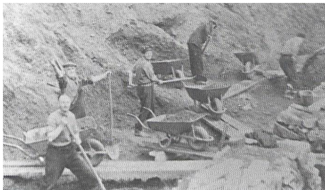
Cliff gang at work helping to stabilize the cliffs. 1961.
