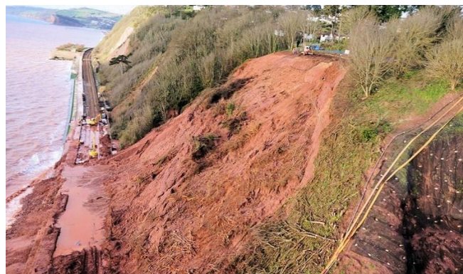
Slope failure adjacent to Parsons Tunnel February 2014.
