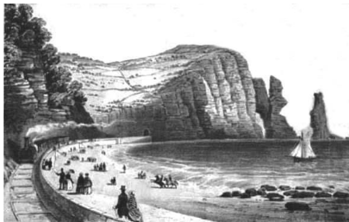
View at Parsons Tunnel.
