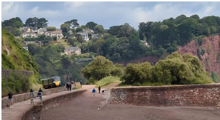
Western side of Sprey Point as it is at June 2024.
