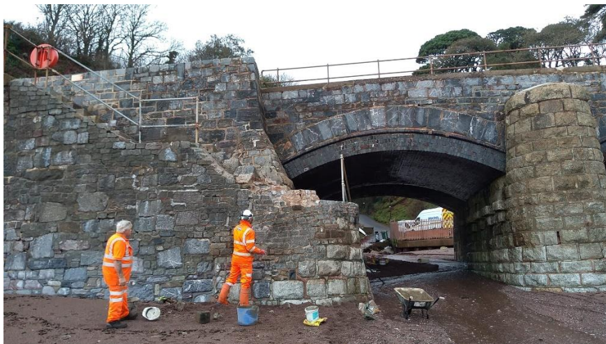
'Orange Army' on repair duties at Smugglers Lane.
