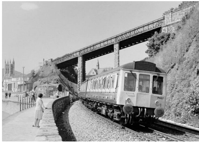
Eastcliff end of the sea wall in 1985 with diesel train heading east.
