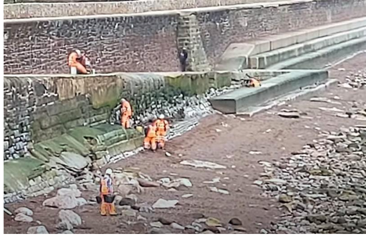
'Orange Army' carrying out repairs. March 2021.
