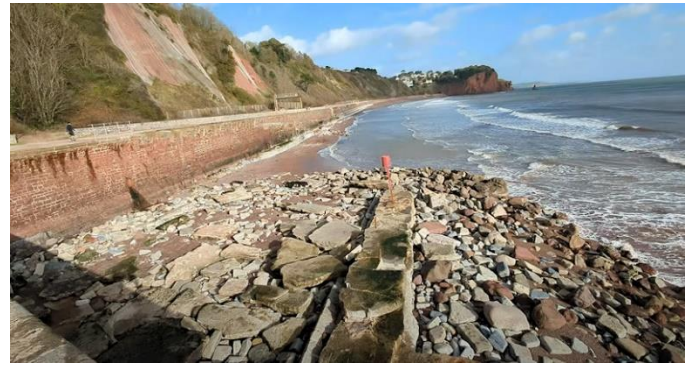
Eastern breakwater at Nov 2023.
