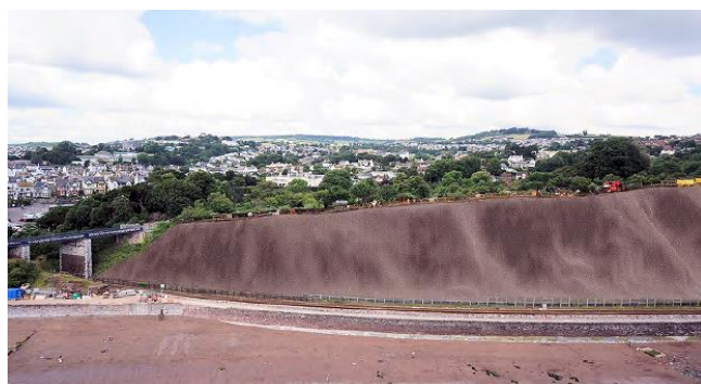
Eastcliff with meshing installed.
