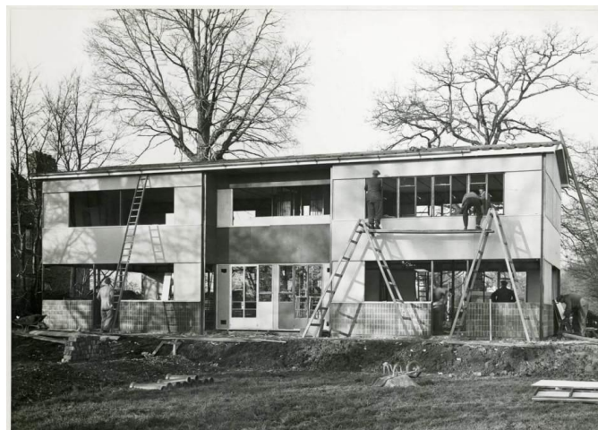
A Howard House under construction in Windsor and Maidenhead. The prefabricated Howard House was designed by architect Frederick Gibberd and produced by John Howard & Co. Constructed using a light steel frame clad with asbestos panels.
