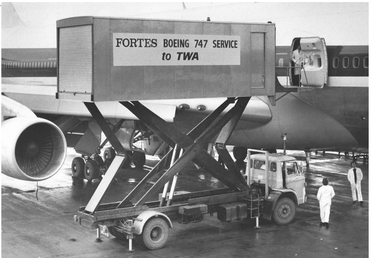
Above: This wagon is at the airport and working for Fortes food group, fitted with a scissors-lift as a support vehicle on the TWA 'Jumbo Jet' service.
