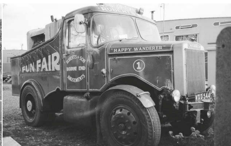
Above: Scammell Highwayman ballast tractor, VXD 544 (London, 1958-59), M2084 in the Pickfords fleet is seen with a draw-bar low-loader trailer, with four-in-line bogies, awaiting its next load, and as 'Happy Wanderer', with amusements operator, Roberts & Son, of Bourne End, Buckinghamshire, its usual ballast box body extended at the rear to accommodate the customary generating set.
