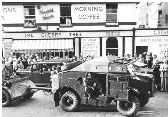
Above: The armed services were represented here with a Morris Commercial C8 Quad field artillery tractor, featuring a canvas top. This identifies it as a 1944/45 build, according to Bart Vanderveen.
